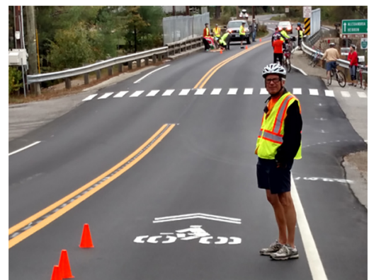
Installation of shared lane marking along West Shore Road in Bristol
